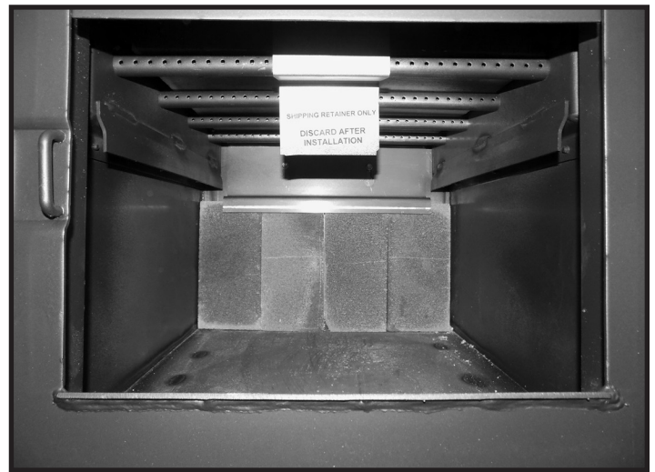
Figure 20: Bricks against rear wall.
