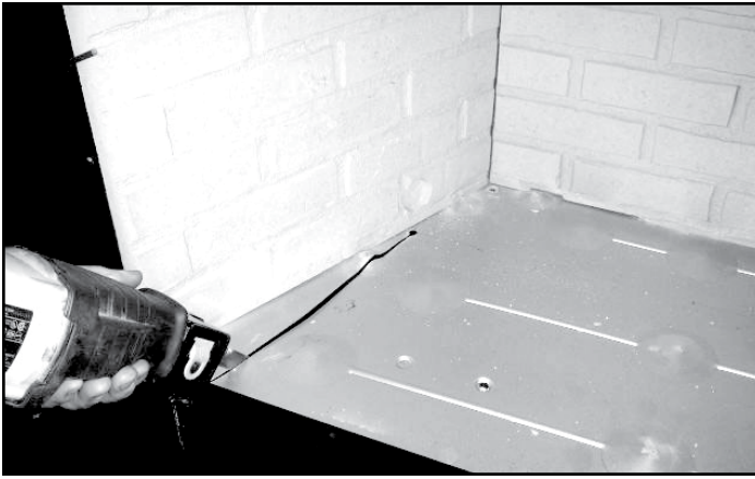
Figure 12.1 - Using a saws-all, cut out the floor.
