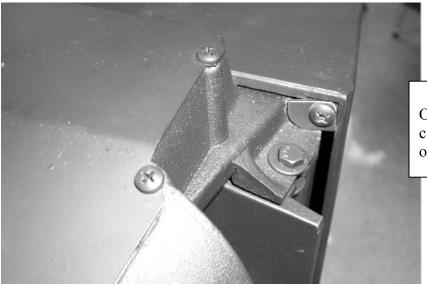
**PHOTO #5** One of the two retaining clips and screws on the back of the façade.
