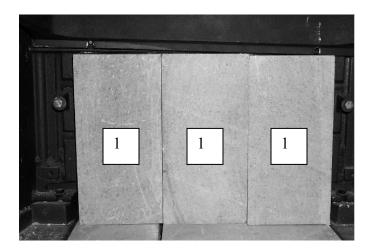
**PHOTO #12** Set three stones vertically against the back of the firebox
