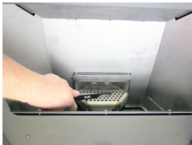
4. Brush away flyash around the fire platform using the brush included with the insert. The flyash will fall into the ashpan below.
