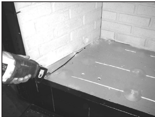
Figure 11.2. Using a saws-all, cut out the floor
