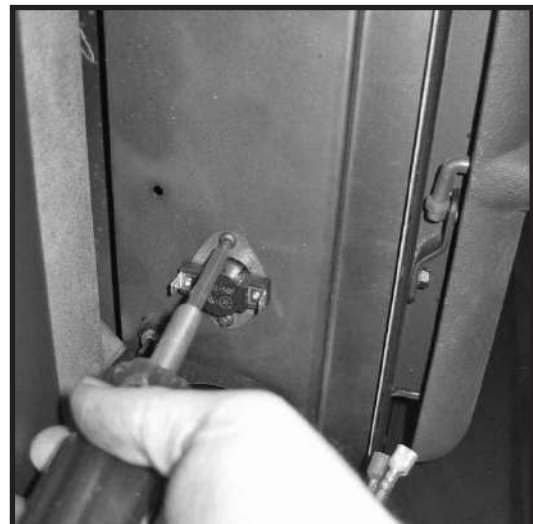
Figure 23: Relocating thermal switch to left side.
