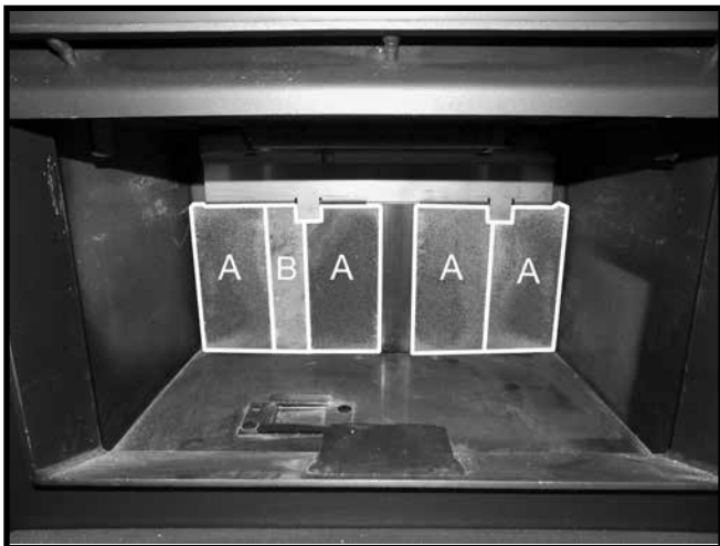
Figure 20: Left side rear wall A and B brick placement.
