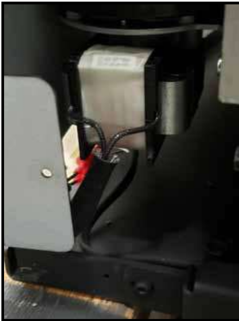
Figure 14: Wire Location LHS.
