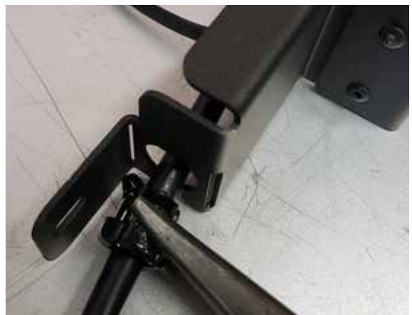
Figure 18: Left Strain install.
