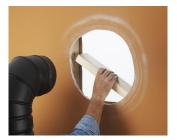
3- You must first secure the wall thimble into the exterior wall surface. Then, do the same inside and fasten the trim plate.
