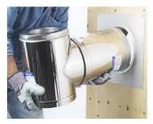
5- You can now install the wall support. Simply slide the wall support up to the tee, ensuring that the adapter on the support engages with the female coupler on the bottom of the tee. When the wall support is level and properly positioned, you can use lag bolts to secure it into the wall studs. To complete the installation, install an insulated tee plug below the wall support.
