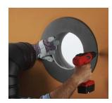
4- Then, from outside the building, slide a short chimney length (attached to the tee) through the wall thimble. The chimney must extend at least 3 inches into the living space where it attaches to the stove pipe.
