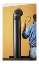
2- Once the opening completed, you need to frame in the area to allow for the installation of a wall thimble. A wall thimble is not required for installations through concrete walls.
