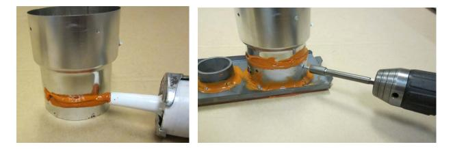
3 Apply a bead of high-temperature RTV silicone to the chimney liner. Insert the chimney liner into the slip connector and secure using (4) sheet metal screws. Apply additional RTV silicone to the area around the connection to ensure an air-tight seal.
