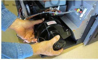
4 Remove all dust and debris from the convection blower. NOTE: Take care to prevent damaging the impellers.
