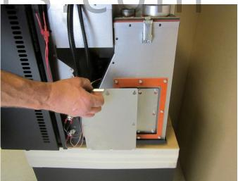
3. Loosen the 8 screws holding the exhaust duct cover in place (11/32" nutdriver). Remove the exhaust duct cover by sliding it up and off the studs (the gasket will remain in place).
