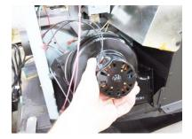
4. Remove all dust and debris from the convection blower. **NOTE: Take care to prevent damaging the impellers.**
